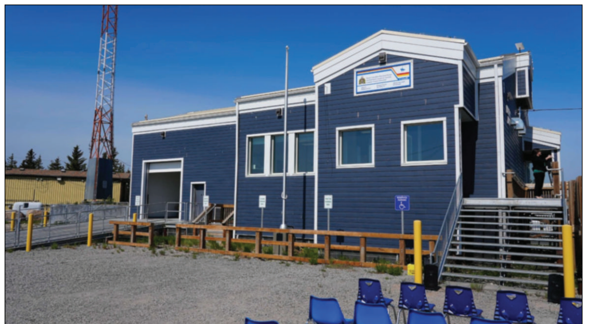
Whati has a new RCMP detachment facility after three years of construction. Photo courtesy RCMP
