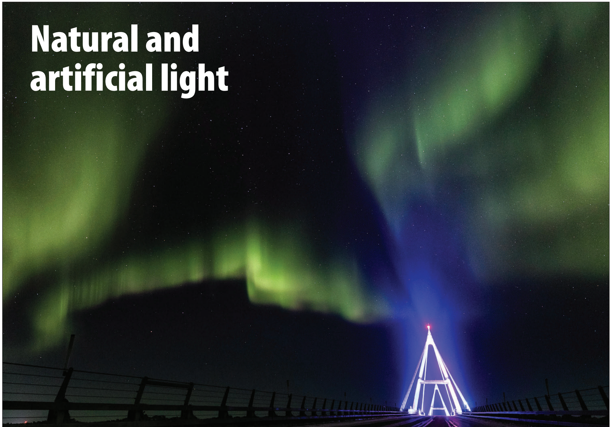
The wavy green Northern lights complemented the lights illuminating the Deh Cho Bridge on a clear night in late March near Fort Providence. Photo courtesy of Thorsten Gohl
